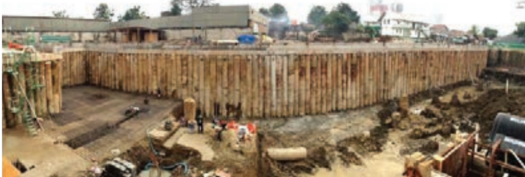
Secant Piles , Proyek Puri Matahari Tower (2013)
