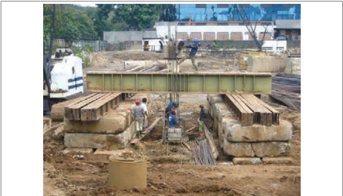
Tes tarik, Proyek Altira Business Park (2012)
