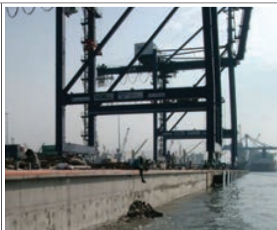
Hasil Diaphragm Wall Proyek JICT Tanjung Priok (2003)
