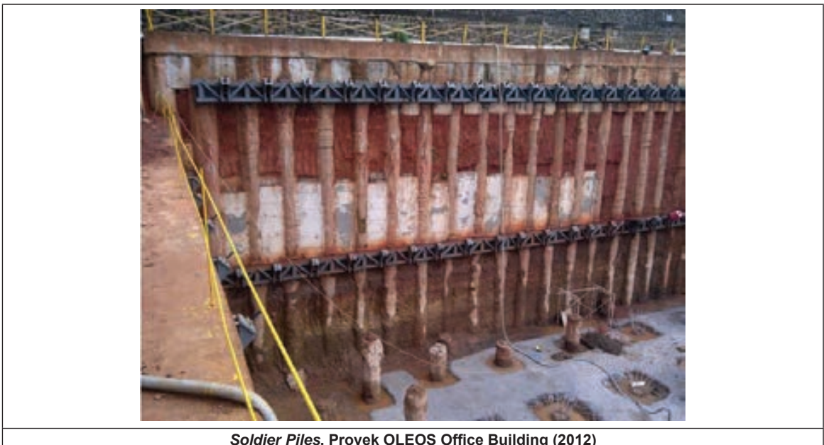
Soldier Piles , Proyek OLEOS Office Building (2012)
