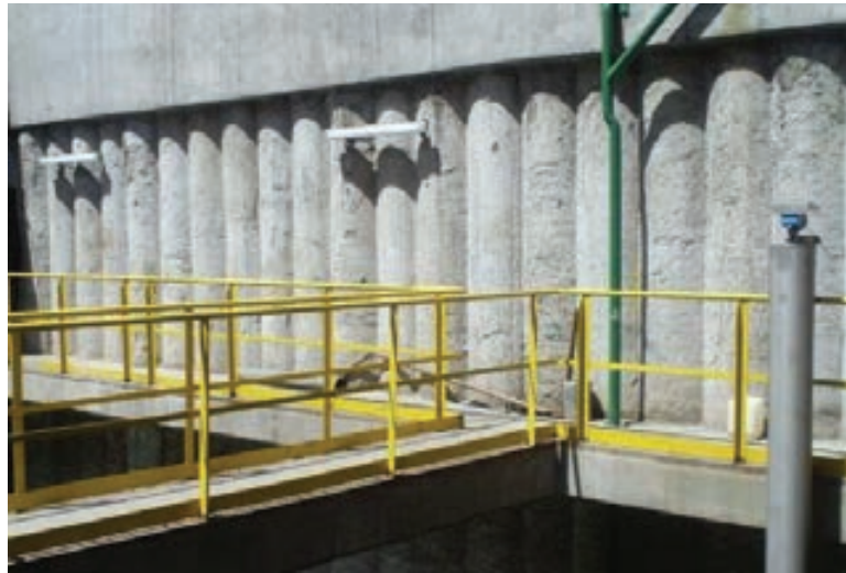
Secant Piles , Proyek Scale Pit Krakatau Steel (2011)
