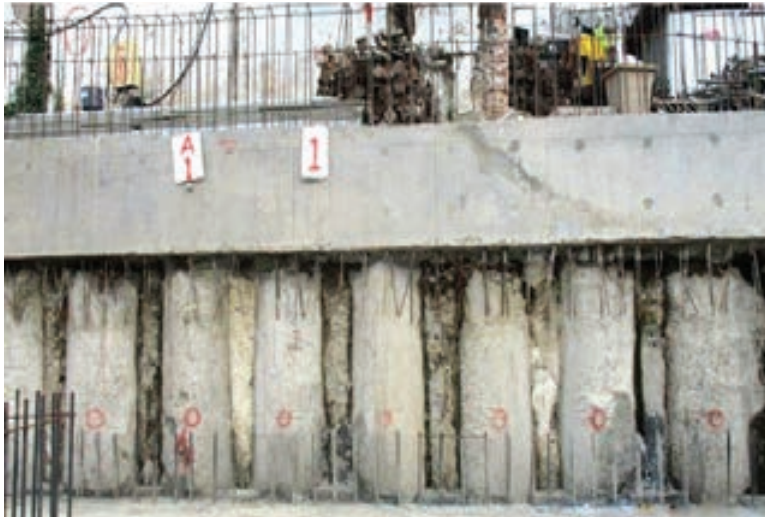
Contiguous Piles, Proyek Praxis - Surabaya (2014)
