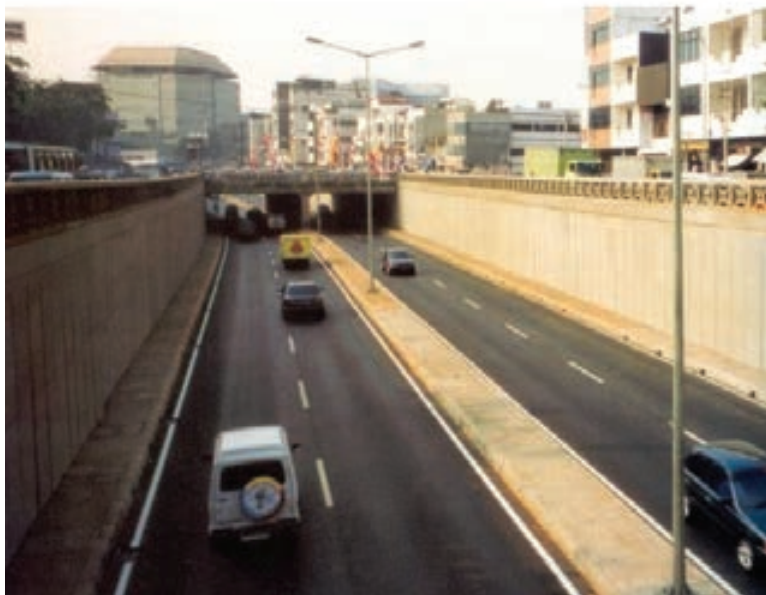
Diaphragm Wall Precast Proyek Underpass Tanah Abang (1996)
