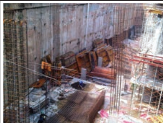
Hasil Diaphragm Wall Proyek Tempo Scan Tower (2009)
