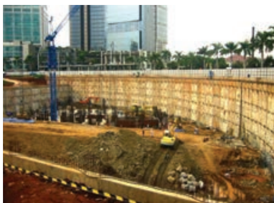
Hasil Diaphragm Wall Proyek Ritz Carlton Hotel - Mega Kuningan (2003)
