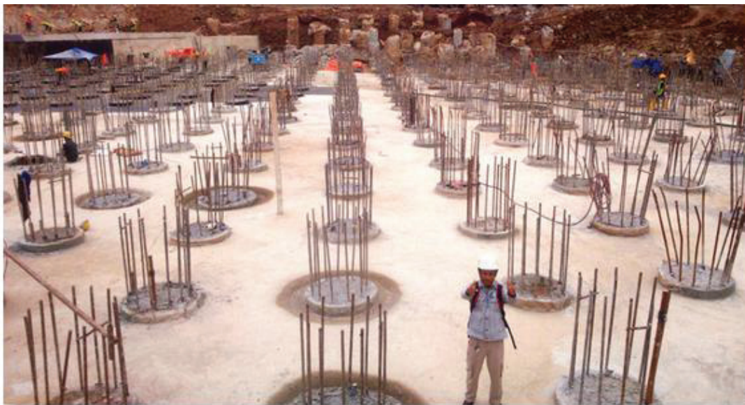
Hasil Tiang Bor ( Bored Pile ) Proyek Icon Complex (2013)
