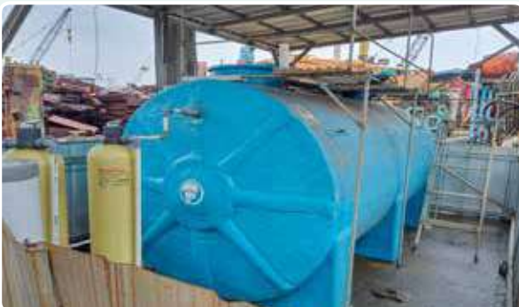
Pengoperasian IPAL berkapasitas 8 m 3 /hari WWTP operation with a capacity of 8 m 3 /day
