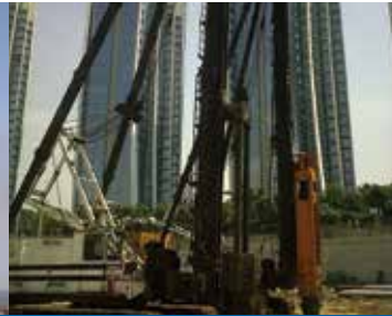
Diesel & Hydraulic Hammer
